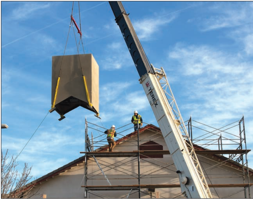
Two new cupolas are placed atop the MPB, one is to disguise a cell tower
